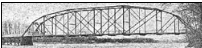
St. George's Island Bridge (Zoo Bridge) was built in 1908
