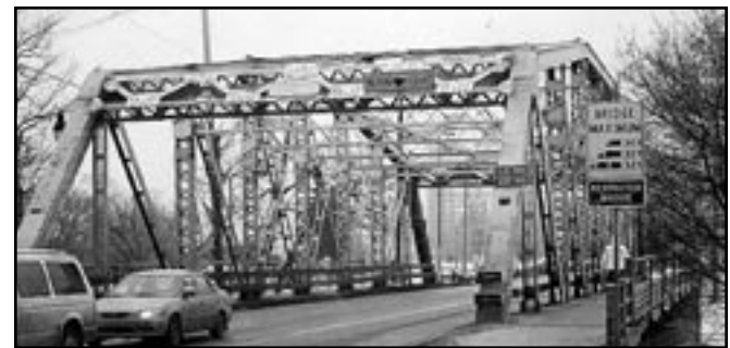
The 9th Avenue Bridge from Inglewood to downtown.
